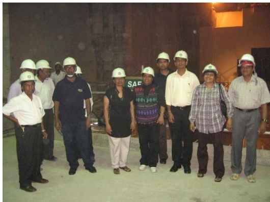
Upper Kothmale Power house –inside the Tunnel Base
